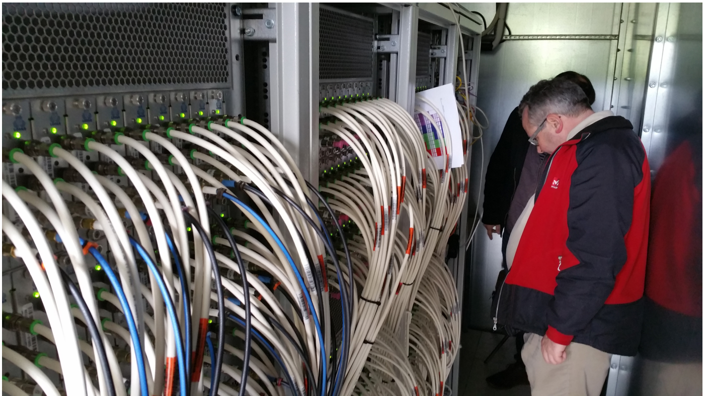
The LOFAR receiver shack, a 20' sea container. These racks contain the digitizers for all the high-band and low-band array elements.
